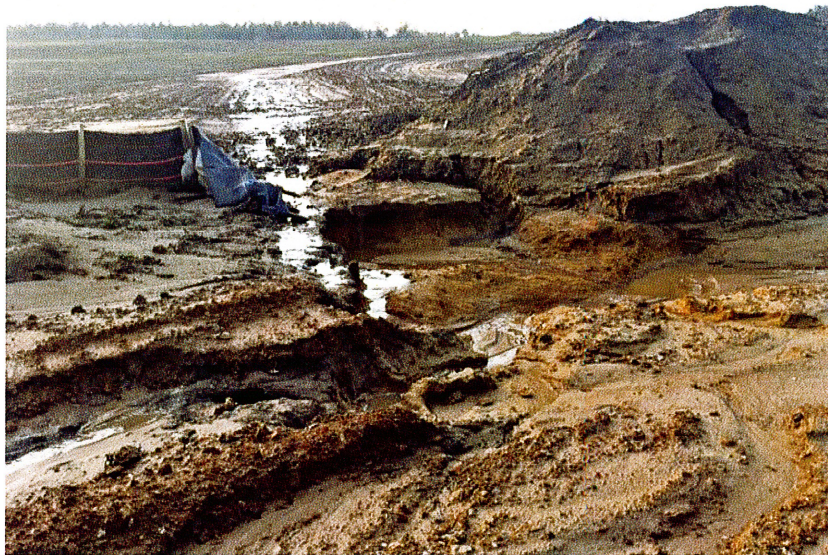
A breached sediment barrier at the mouth of a terrace is a violation of Georgia's Soil and Water Commission's Green Book.
