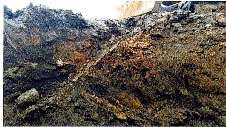
While repairing an irrigation line, Randy Dowdy found jumbled soil deposition. "Even the soil that was saved and put back on my land wasn't segregated."
