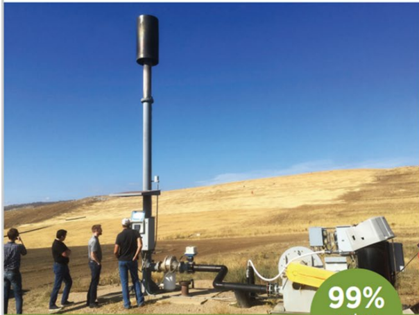
Larimer County Landfill | Fort Collins, Colorado
