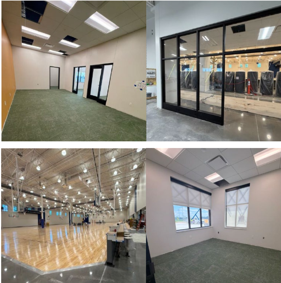
Interior Progress – Classrooms and Gymnasium
