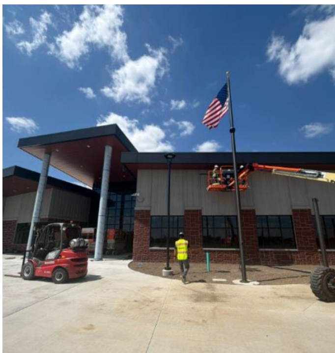
Exterior Progress – Main Entrance
